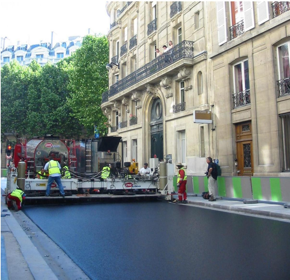
*Machine laid mastic asphalt pavement.*
