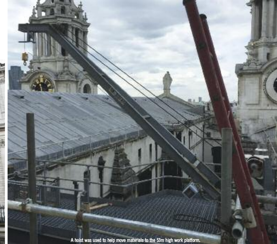
A hoist was used to help move materials to the 53m high work platform.
