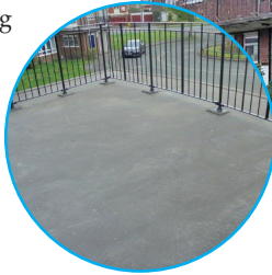
Brindley Asphalt Roofing applied the IKO Permaphalt mastic asphalt system for the Merridale Court project
